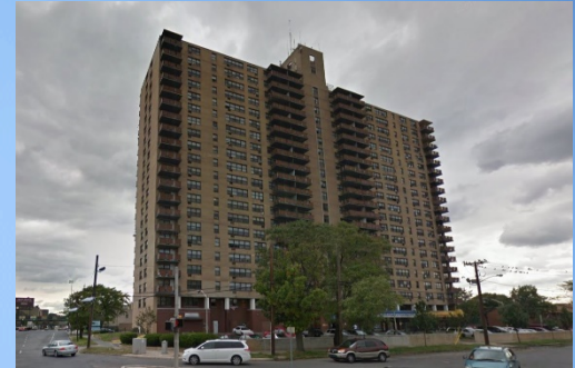
Northgate I Apartments Camden, NJ
